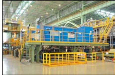
感应炉 Induction furnace
