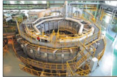
环形炉 Circular furnace
